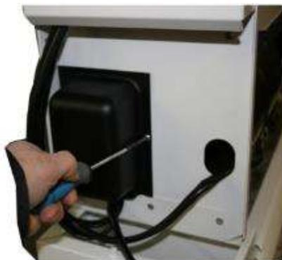
10 Connect power and remote humidostat wires.
